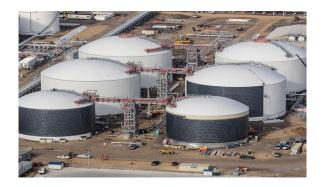
• **Self-supported umbrella roof:** It is a kind of the dome roof tank that has been modified, each horizontal part of which is a regular polygon.
