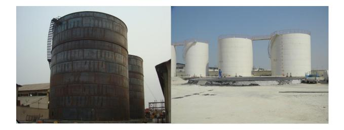
Fixed roof tanks come in a variety of shapes, including domed, conical or canopy roofs. Cone and dome roofs are more common. Operationally, conical roofs are more common, but domed roofs are more robust. In the next section, each of these tanks is described.
