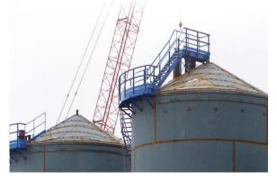
• **Self-supported dome roof:** This type of roof is spherical and relies only on its environment. Figure 5 shows an example of a tank with a domed roof.
